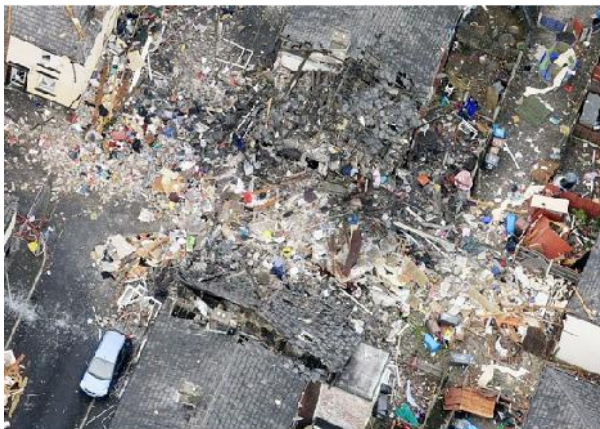
Figure 3: Devastation caused by a recent gas explosion (Telegraph, 2012)
