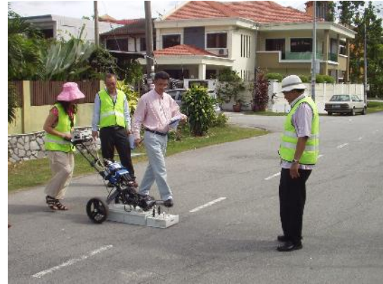
Figure 10: Course participants demonstrating Use of GPR for utility detection
