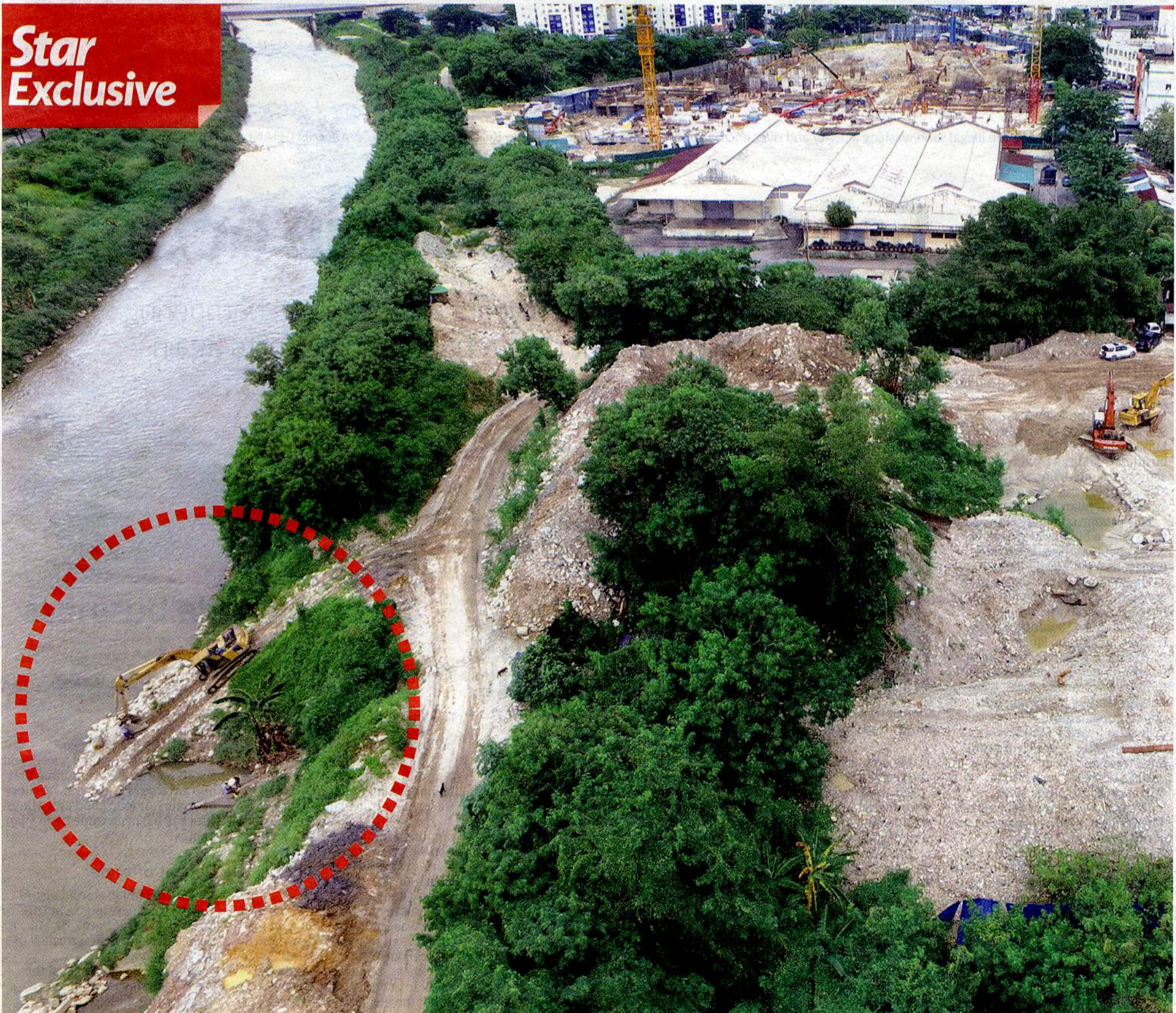
Sneaky activities: An aerial view of the sand-washing operation near 5th Mile off Jalan Kelang Lama found to be active again after two years. An excavator is also seen encroaching into the riverbank. — FAIHAN GHANI/The Star
