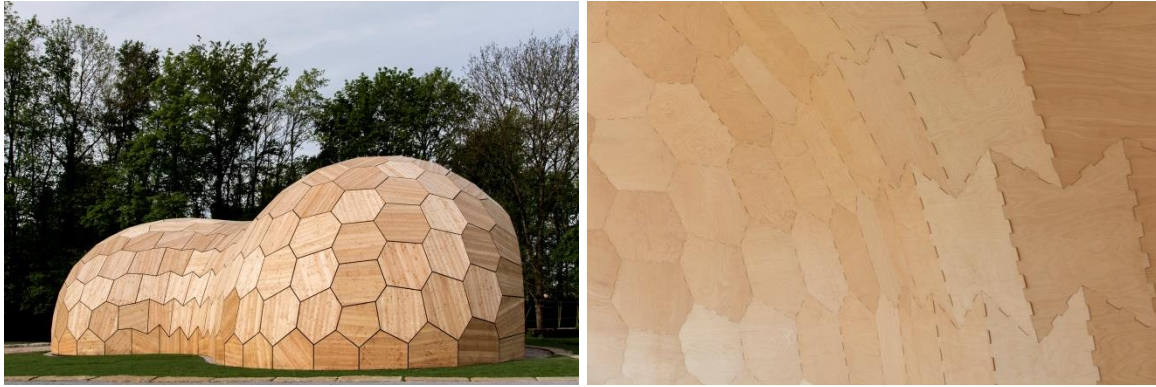
Fig. 1 a) Exterior view of the pavilion b) Plate structure ©ICD/ITKE/IIGS, University of Stuttgart.
