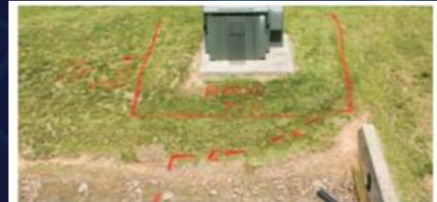
Example of electric transformer, hand dig zone, corridor, lateral
